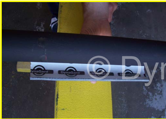
To install, confirm that the DynaGard fits snugly onto the pipe to be protected
