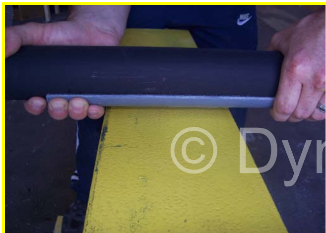
Place the DynaGard under the pipe, center it over the support and pull up
